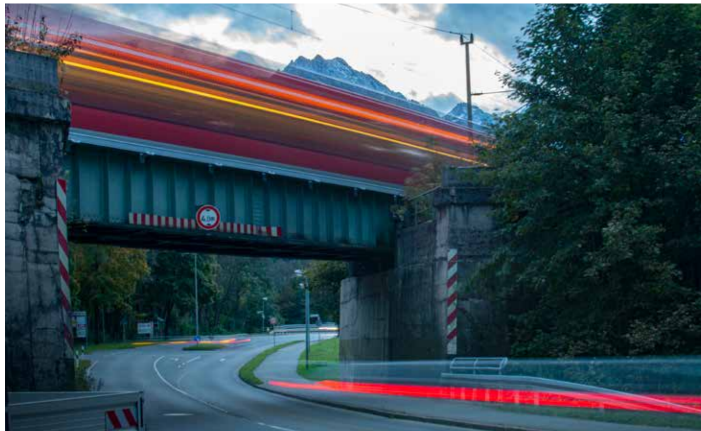
After the installation
