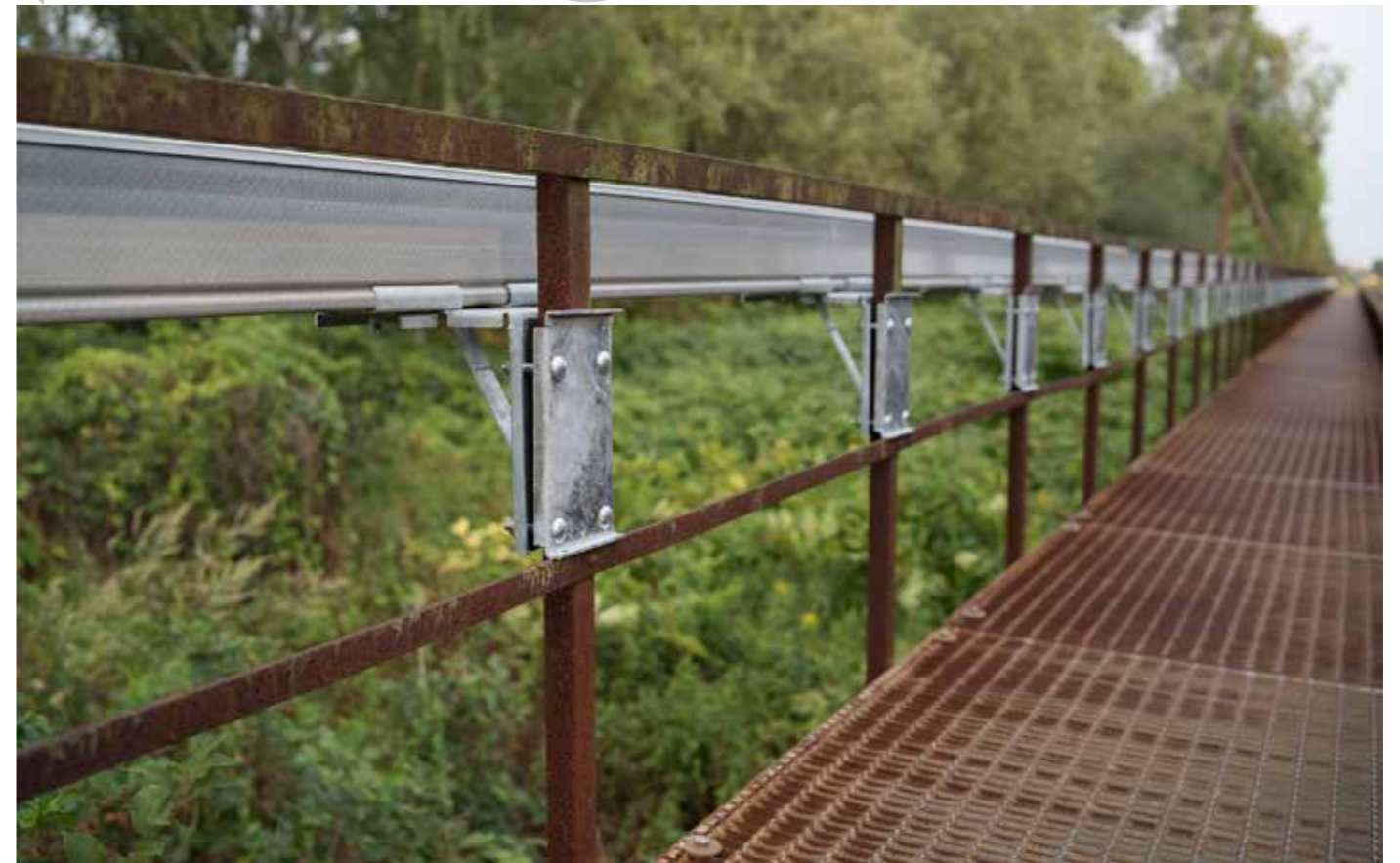
Positioning of round head screw can be done from both sides
