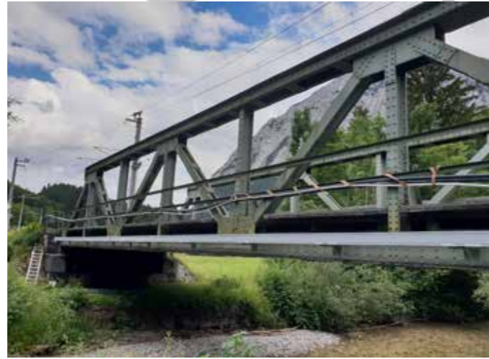
After the installation
