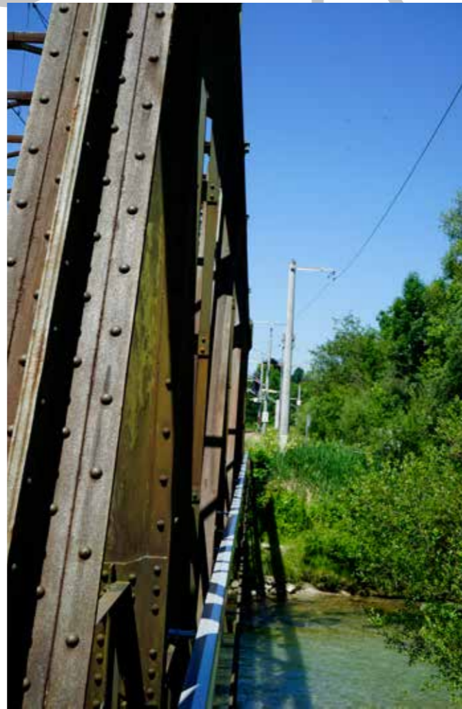
After the installation
