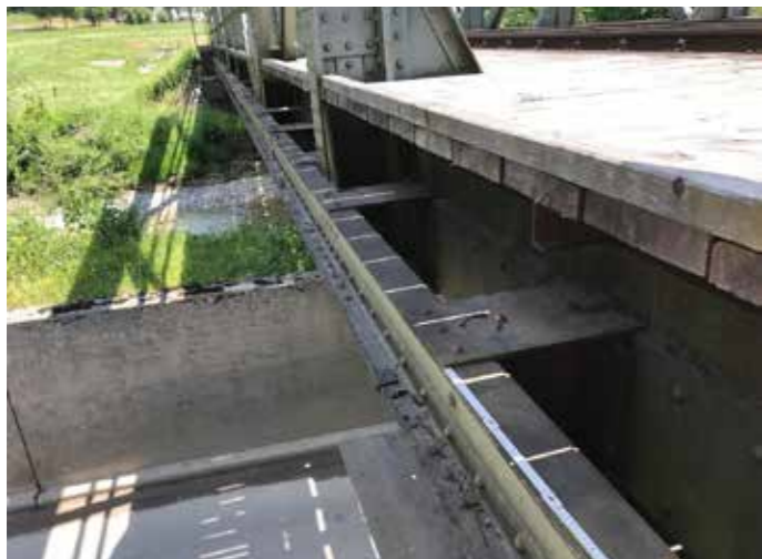
After the installation
