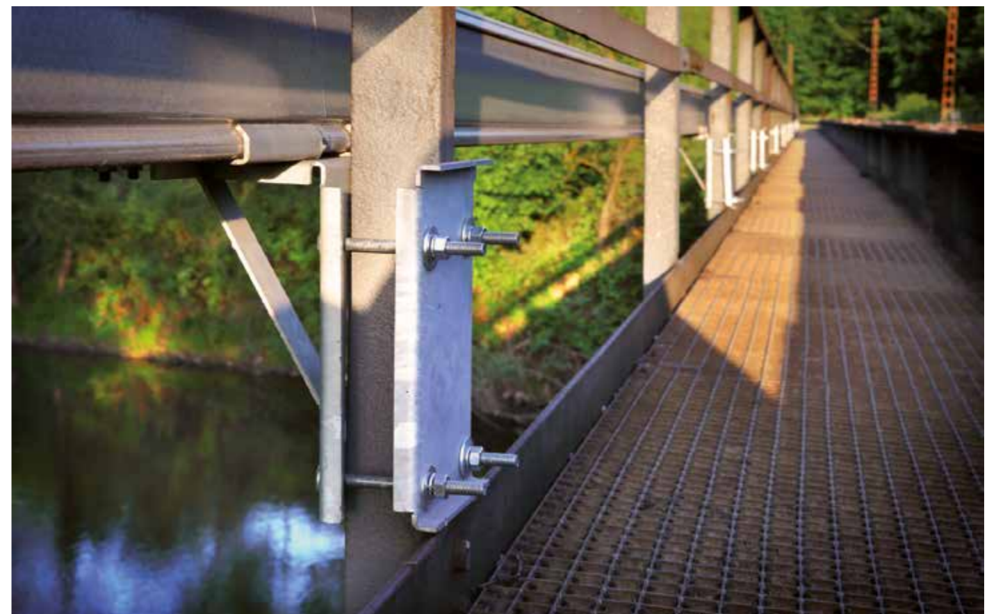
Positioning of round head screw can be done from both sides
