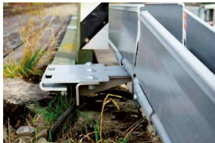
After the installation
